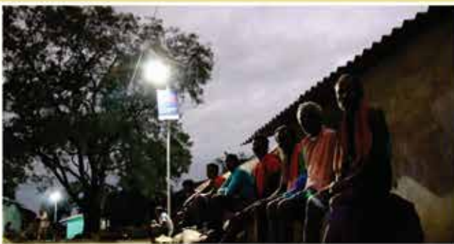
Solar Street Light for Community Usage at Patramunda Village
