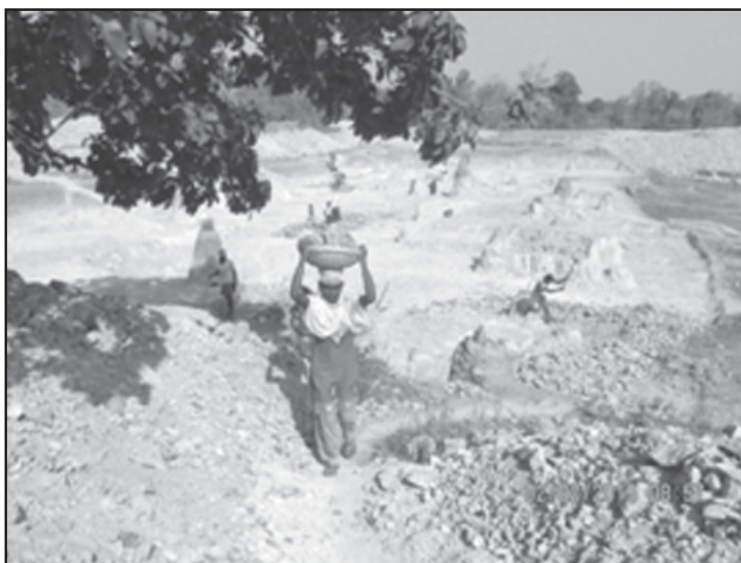
MGNREGS work under progress in Godfula village, Kuliabandh GP, Nuapada District
