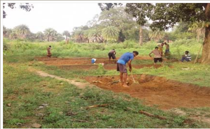
MGNREGS Work in Progress Kurkunda GP, Malkangiri Block Under EU Project
